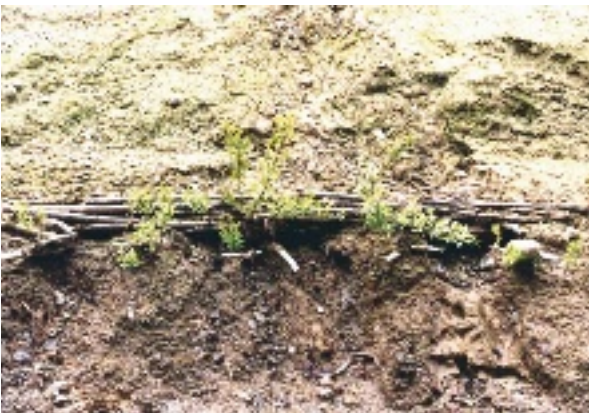
Photo 3 Clayonnage Photo F. REY, 2002
